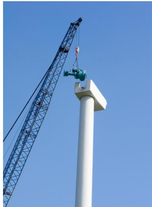
**Fig. 1-Wind Turbine Gearbox Installation**
